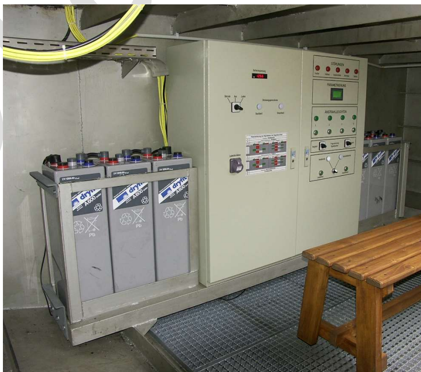
Figure 3 - Installation of Gel batteries in a signalling float
